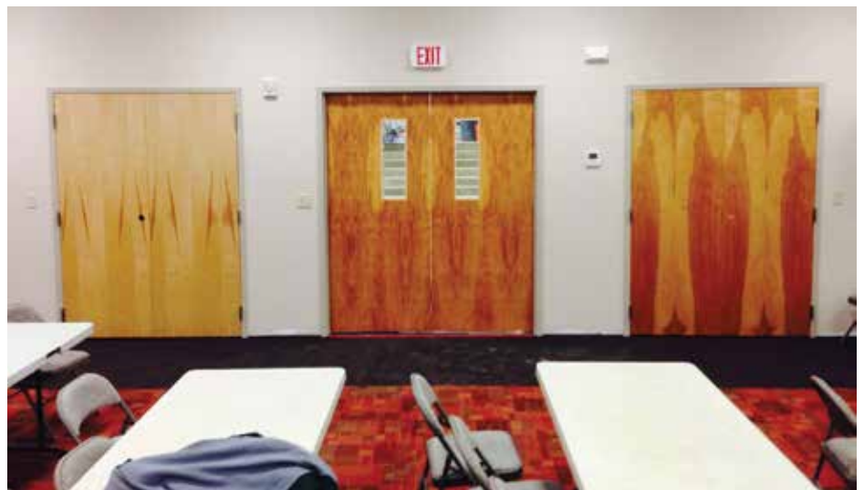
Each pair of these doors met the architectural spec for pair-matched rotary white birch. The architect rejected the three sets because of their combined visual incompatibility.
